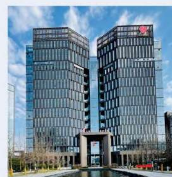
Construction service center in Hangzhou
