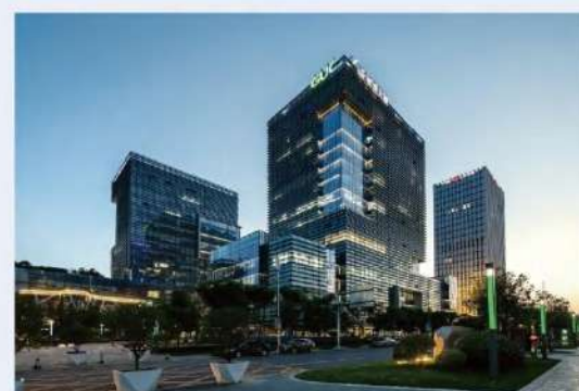
R&D and sales center in Nanjing
